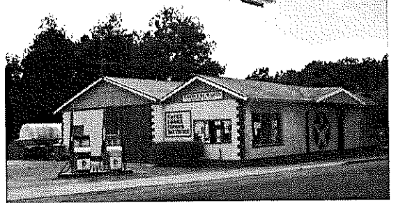
Caltex Service Station.
